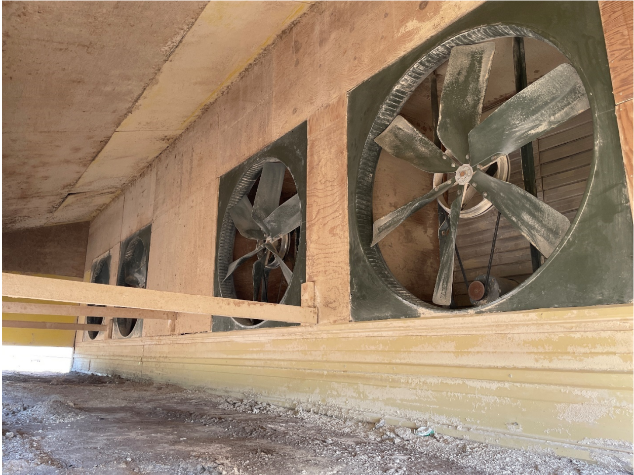
IMG_1403 showing the ventilation fans for barn 25 on the north side of the building. (Note there are not ventilation fans on the south side of the building).
